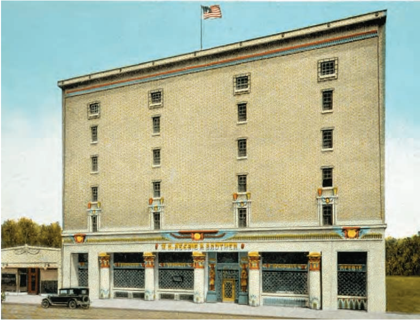
Plate xxxix (a) W. C. Reebe & Brother, Inc., warehouse and general offices, 2325–33 N. Clark Street, Chicago, IL (Chicago Historical Society, I CHI-35525/G81:108.1).
